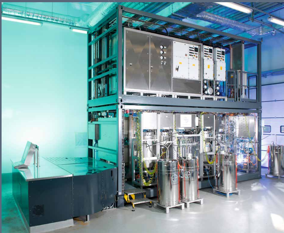
— World's first pilot plant composed of interoperable modules.
